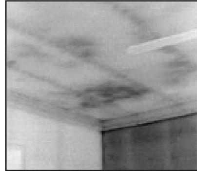
Figure 8: Wet ceiling insulation
